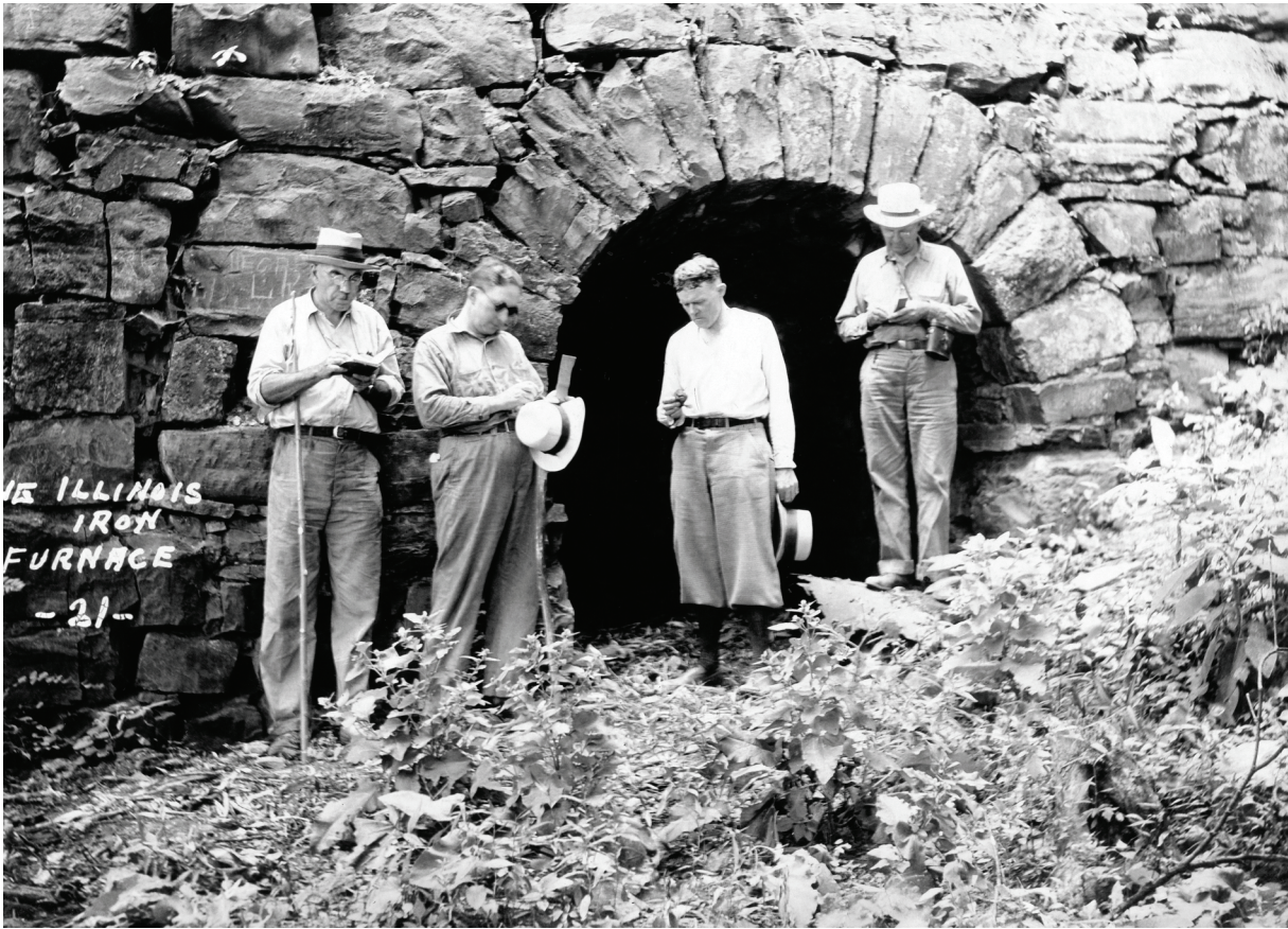
The explorers view the remains of the Illinois Iron Furnace, built between 1837-1839.
